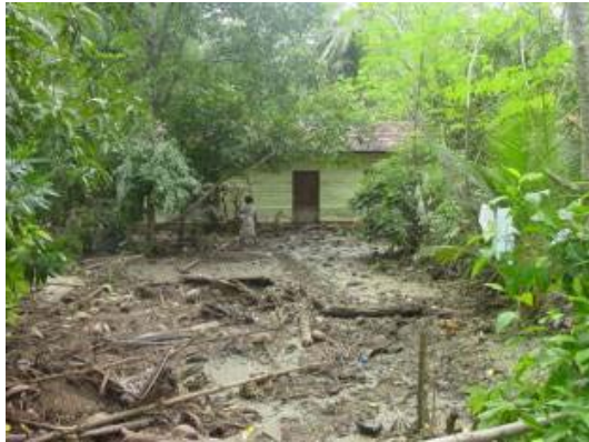
Damaged Home Garden in Wanduruppa
