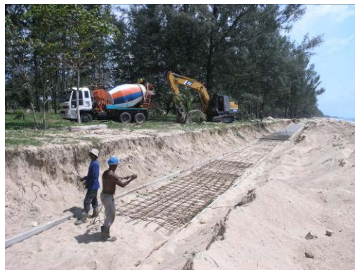
Sea wall construction at Had Tay Muang (courtesy WI Thailand)
