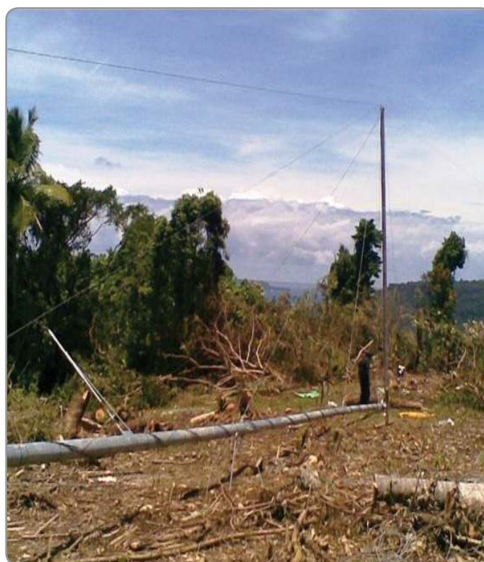
Figure 12: Wind monitoring mast installation in Port Olry
