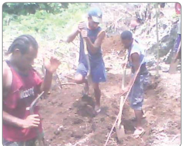
Figure 11: Digging the trench for the Talise hydropower system (Photo taken in November 2011)
