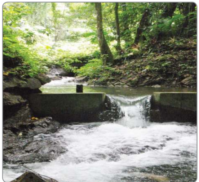
Figure 10: The weir – Photo taken in 2010
