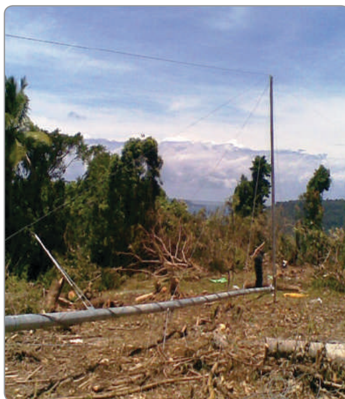
Figure 12: Wind monitoring mast installation in Port Olry
