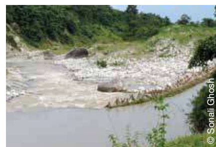
Step 6: Prevention of floods and channelizing the Subankhata River in the upper catchment.
