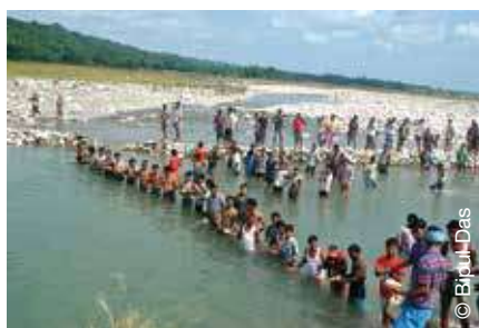
Step 2: Construction of Dong Bundhs before the onset of the dry season (Dec-April).
