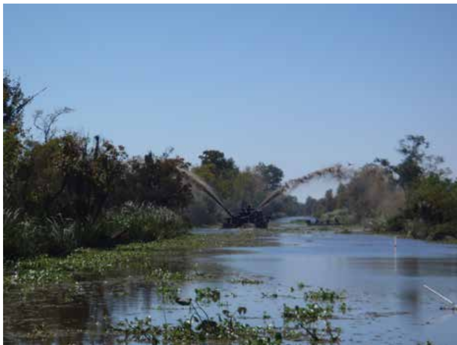
Figure 6: Spray dredge distributing sediments to sides of a canal.
