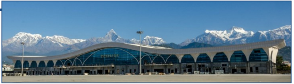
The Pokhara Regional International Airport in Nepal is scheduled to start operations from January 2023. Photo: Civil Aviation Authority of Nepal
