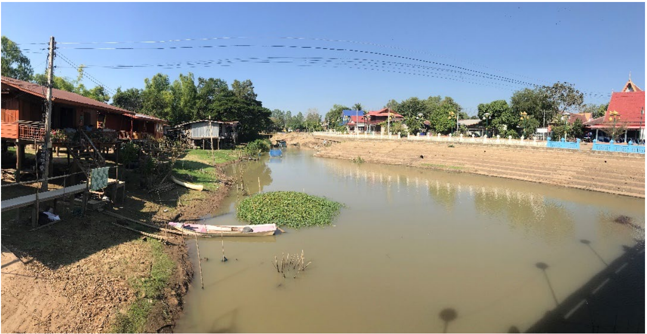
Figure 5 Traditional house on stilts opposite concrete bank reinforcements in Kong Krailat District
