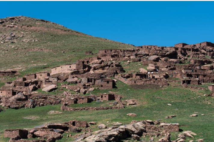
Dry stone walls and buildings in High Atlas, Morocco © Inanc Tekguç GDF
