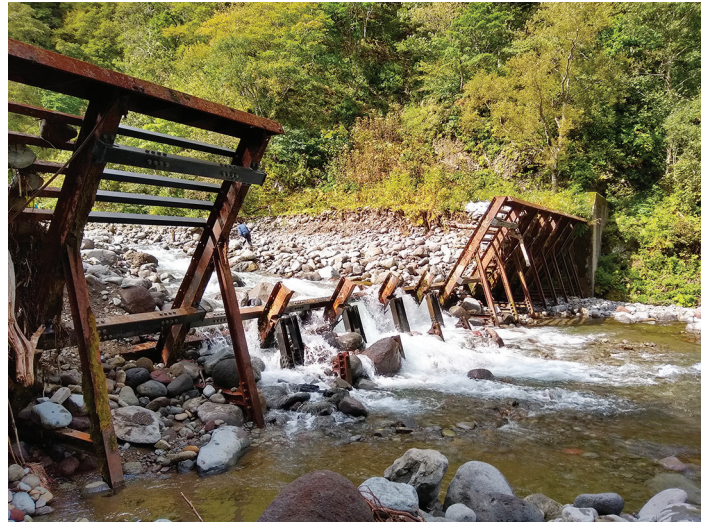
Dam removal in Shiretoko Natural HWS, 2019 Photo: Pete Rand
