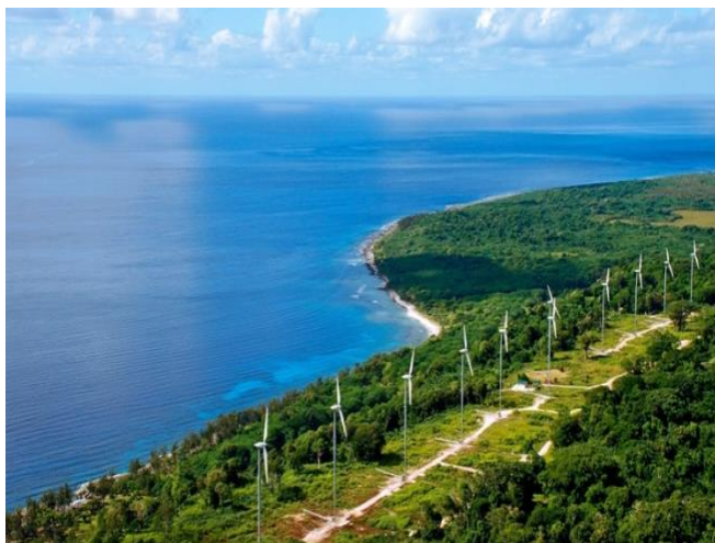
Vanuatu's only large-scale onshore wind generation installation at Devil's Point near Port Vila, Efate island. Source: VERGNET, CC BY-SA 4.0, https://commons.wikimedia.org/wiki/File:Centrale_%C3%A9olienne_Vergnet_Vanuatu.jpg .
