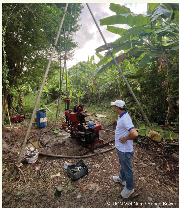
Installing groundwater arsenic monitoring well in An Giang, Viet Nam
