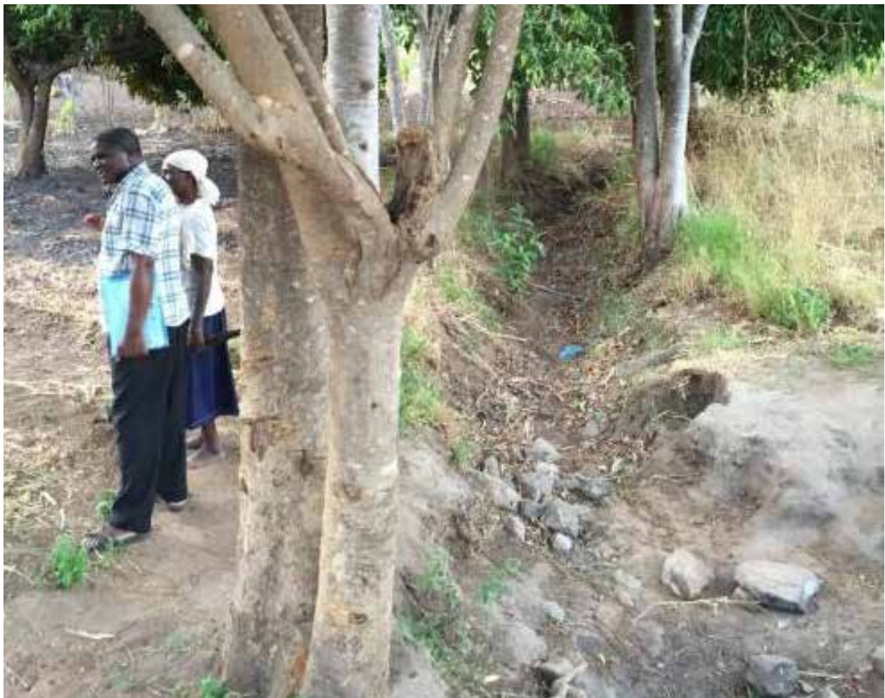
Figure 12 | River- and stream-bank restoration in Machinga District
