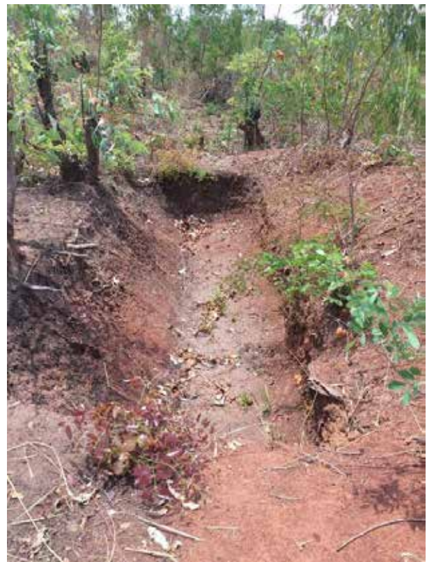
Figure 10 | Examples of soil and water conservation interventions in Machinga District: check dams (left) and infiltration ditch (right)
