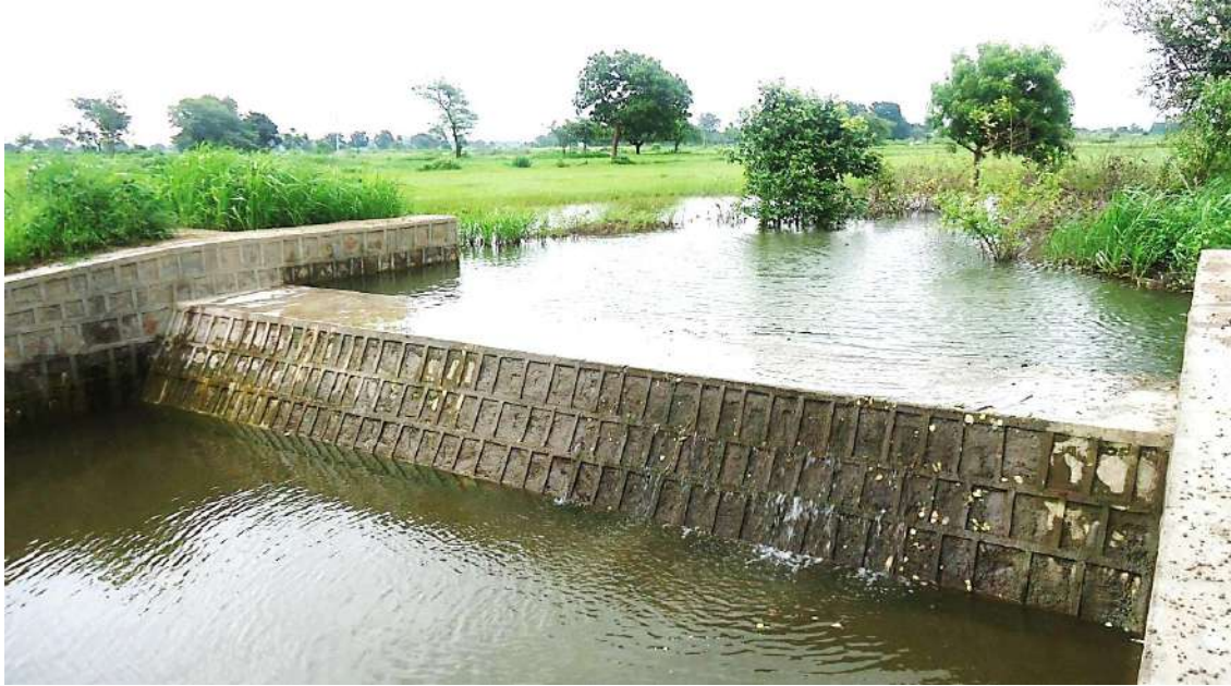
Figure 11: Water storage pond in a farmstead to harvest and channelize rainwater, Datia Watershed, India © Development Alternatives
