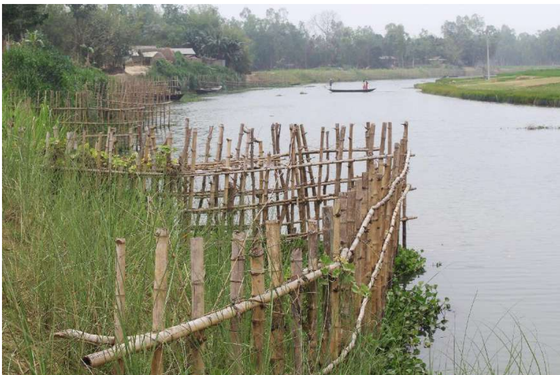
Figure 27: Bank of the Jinjiram river in Namapara Village, one year of year after the riverbank stabilisation activities, with significant reduction in riverbank erosion, Bangladesh ©Oxfam Bangladesh
