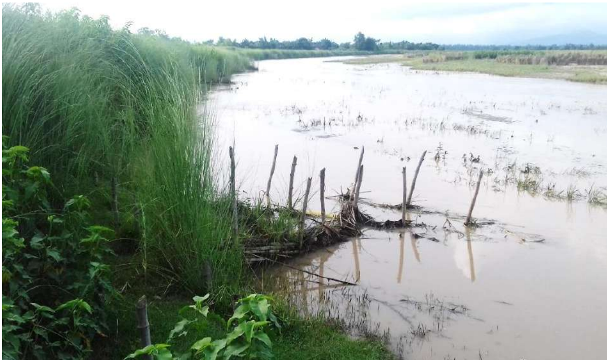
Figure 28: River bank stabilised with the lush green growth of grass, Chaudhar River, Nepal ©Kishan Khadka
