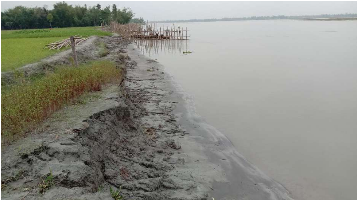
Figure 24: Bamboo-grass based embankments increase sedimentation and reduce river bank erosion on Jinjiram ©Bokhtiar Hossain
