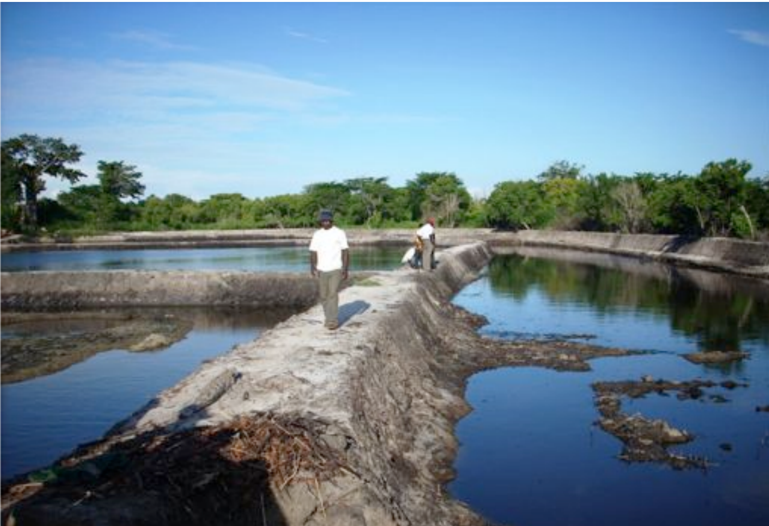
Photo: Chongoleani fishponds under construction, Tanga Region, Tanzania.
