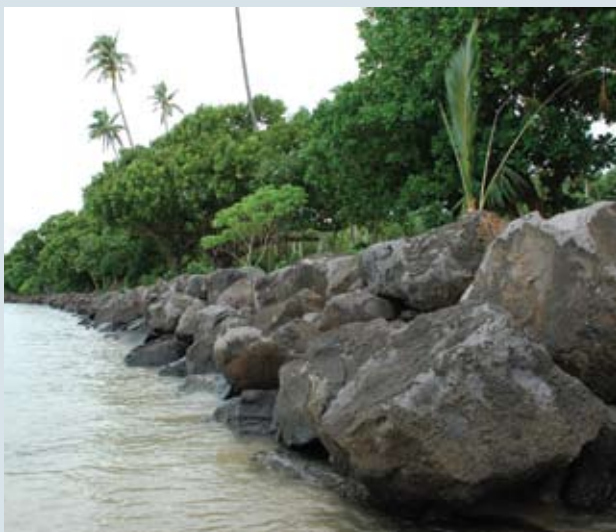
Shoring up the sea front (Vaitapu)
