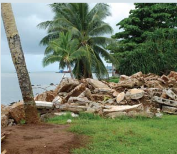
Shoring using building debris (Liku)
