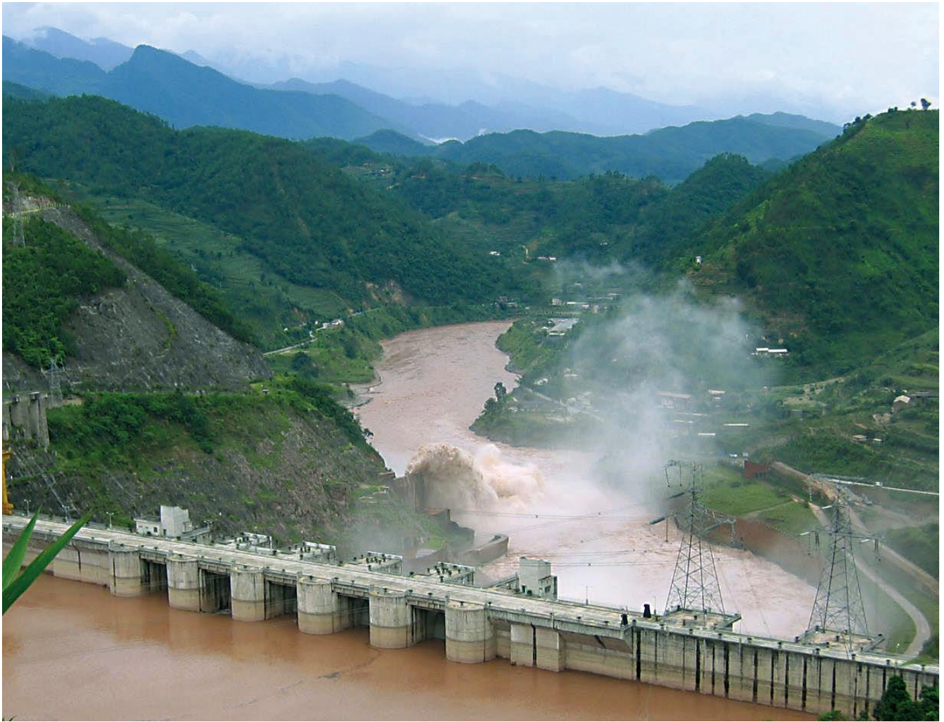
Manwan Dam, the first hydropower project on the Lancang-Mekong River in China. © IUCN
