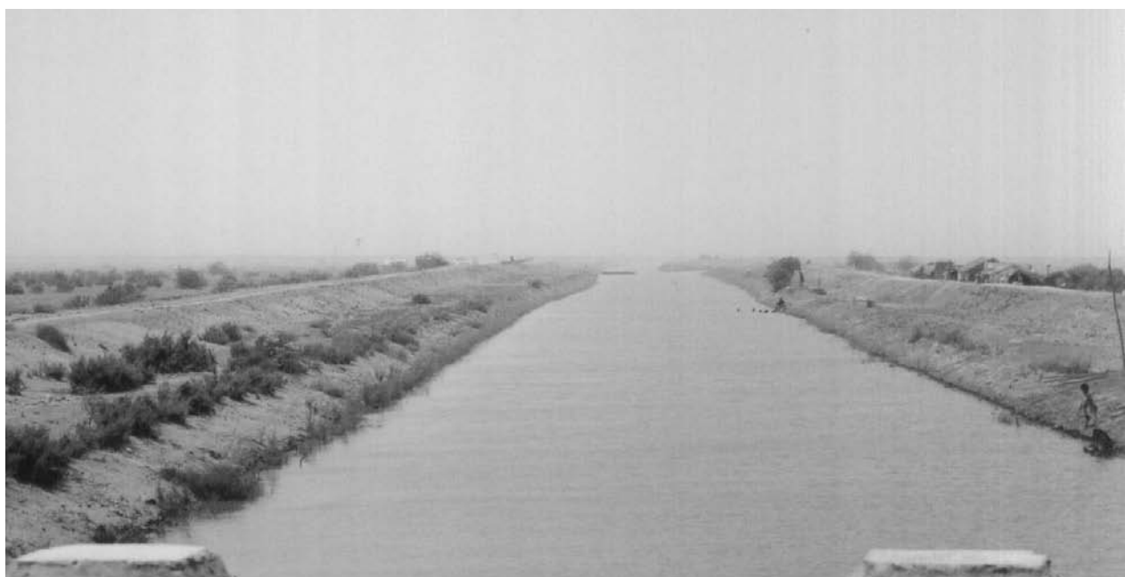
A sub-drain of LBOD project carrying drainage effluents.
