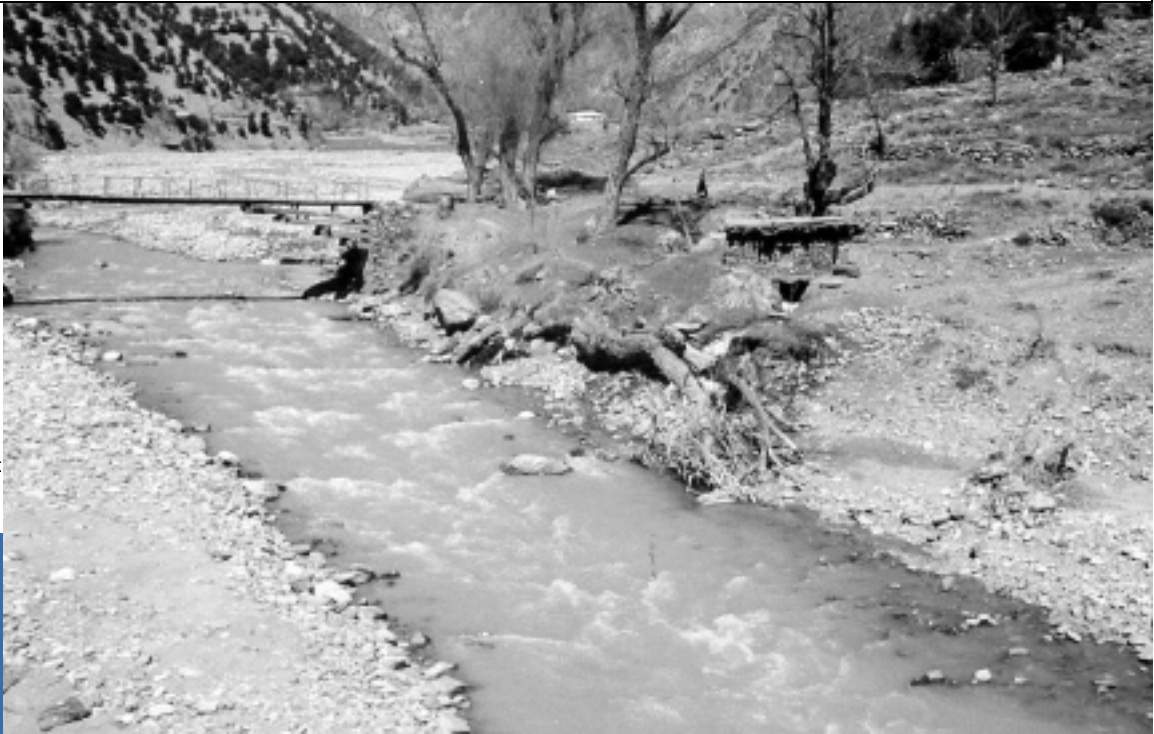
Eroded land – a disturbingly common feature
