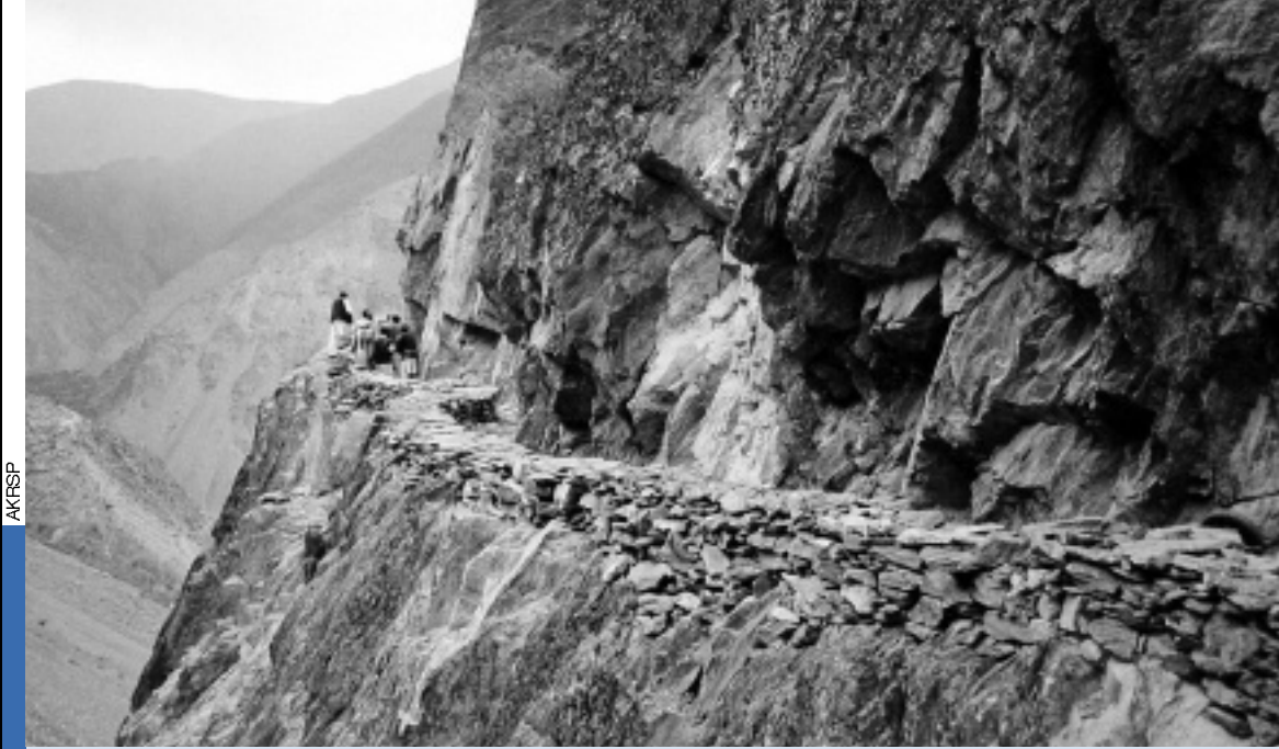
An irrigation channel under construction
