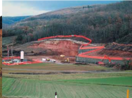
Works on the buffer zone of Selva di Cupigliolo march, 2009
