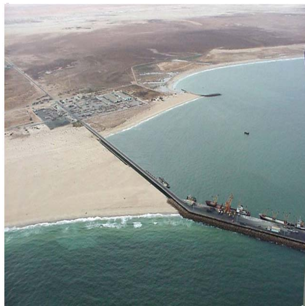
The erosion observed South of the pier at Nouakchott Harbour determines a considerable risk of marine intrusion threatening the urban districts situated below sea level.
