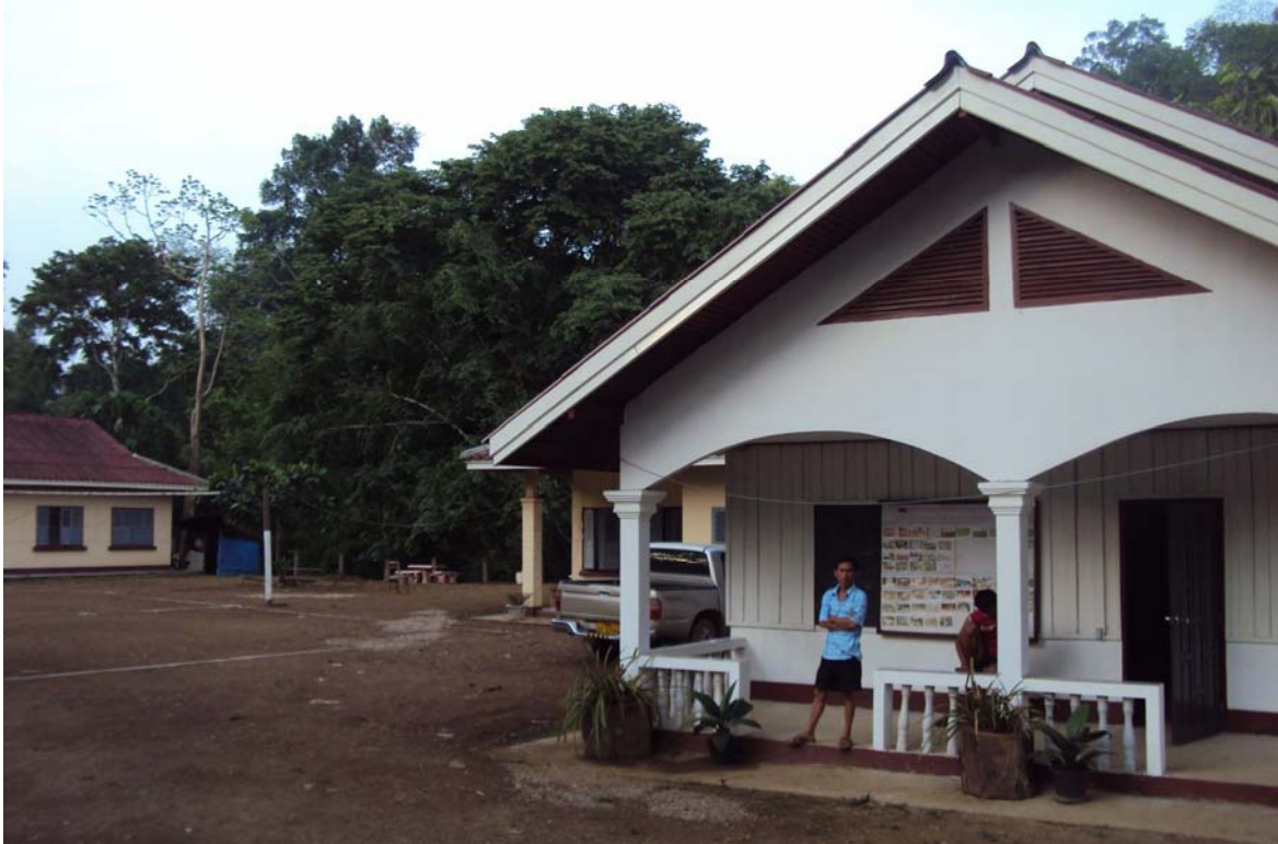
Figure 8. Meeting room and dorms of Nam Phui National Protected Area, funded by the Provincial Agriculture and Forestry Office.
