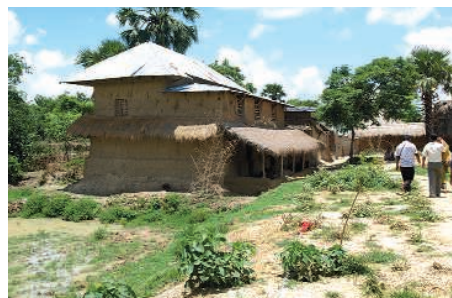
Old and new. Thick mud walls of homes are a time-honored adaptation to scorching heat, while newly dug ponds collect rainwater for irrigation.
