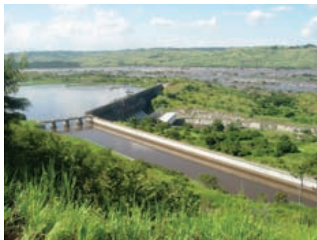
An aerial view of the Inga Dam on the Congo River which, due to lack of maintenance, was running at an estimated 20% capacity in 2006. © INTERNATIONAL RIVERS
