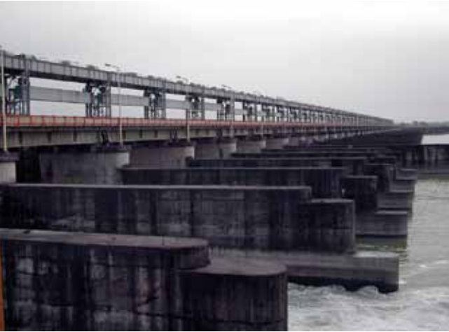
The Tista barrage, an irrigation dam on the Tista River in West Bengal. A series of dams are planned on the river in India, with an estimated total capacity of 50,000 MW. © Heok Hee Ng
