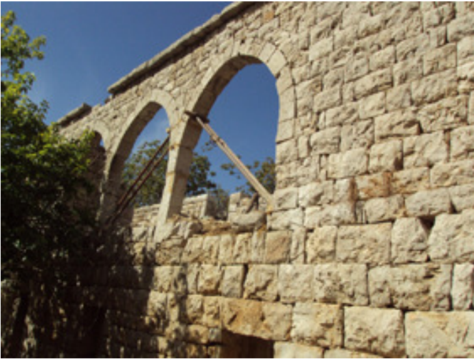
Fig. 5: Old houses being rehabilitated
