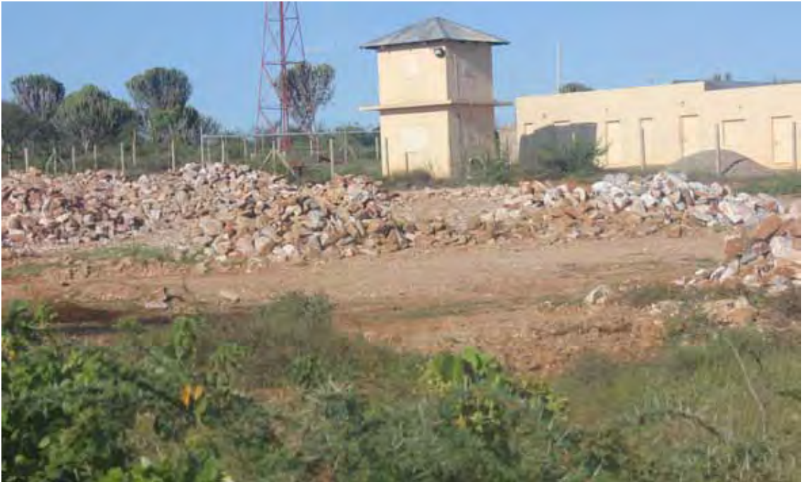
TCL office building at its limestone quarry (photo 4.7).
