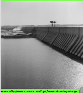
ASWAN DAM ON NILE RIVER
