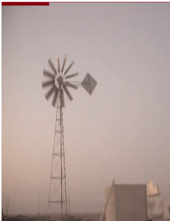
Wind pump installed near Gharo by Karachi University
