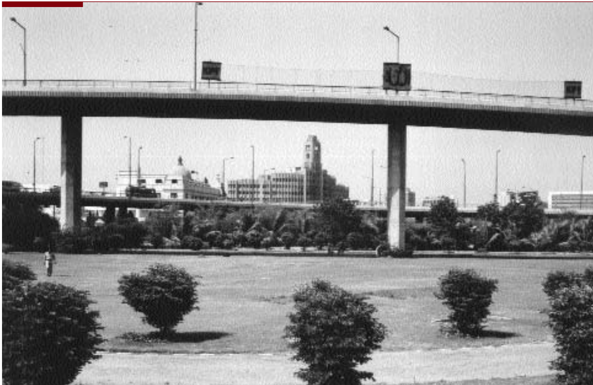
Northern bypass flyover bridge at Karachi, an example of improving infrastructure
