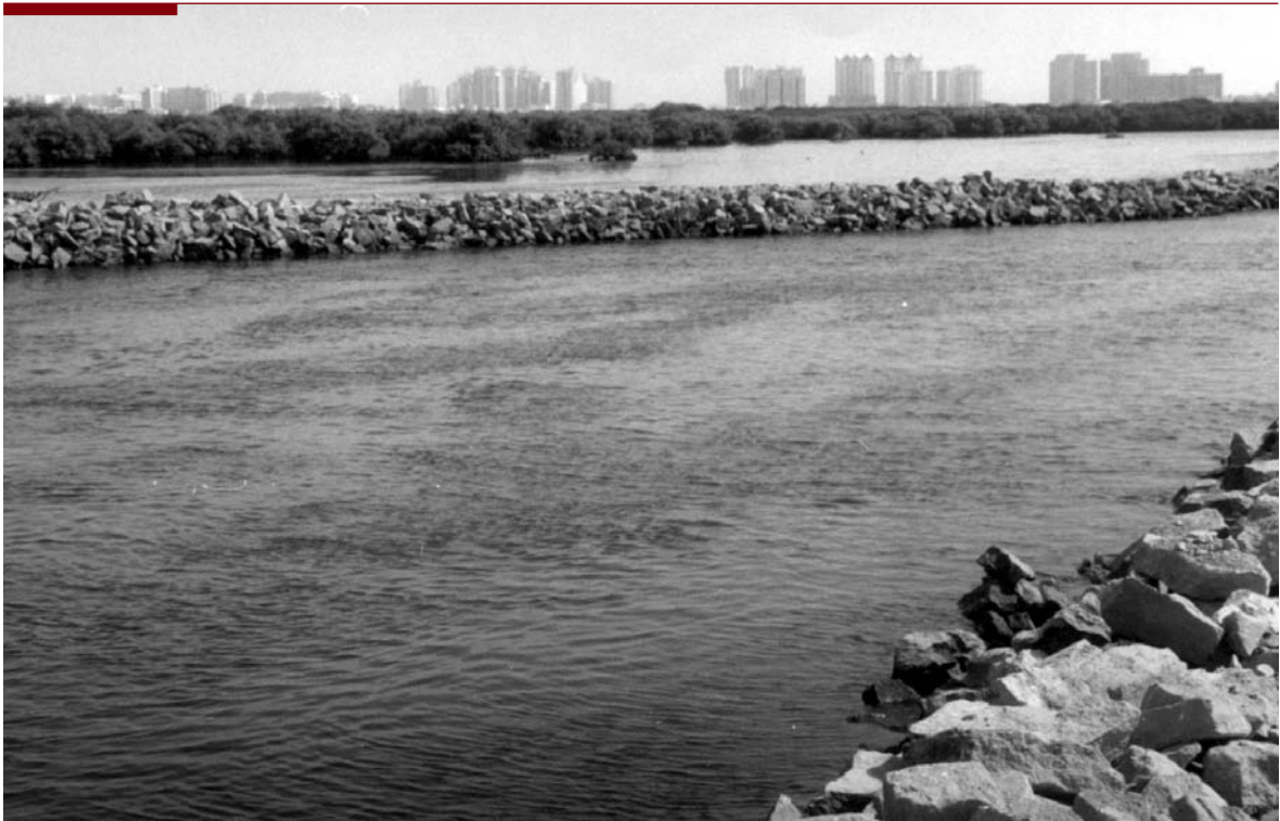
Construction of breakwater is disturbing the ecological balance of the mangroves
