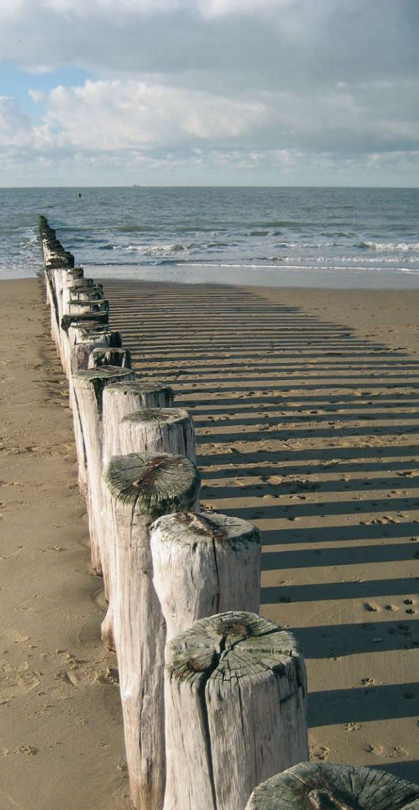
North Sea wave breakers in Zeeland, The Netherlands.
